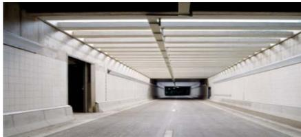
Kinkempois Tunnel (link E25-E40) in Liege, Belgium, using concrete pavement
